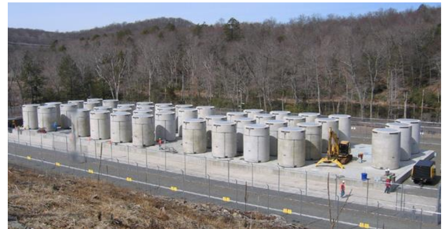
Independent Fuel Storage Installation in the US Source: US DOE
